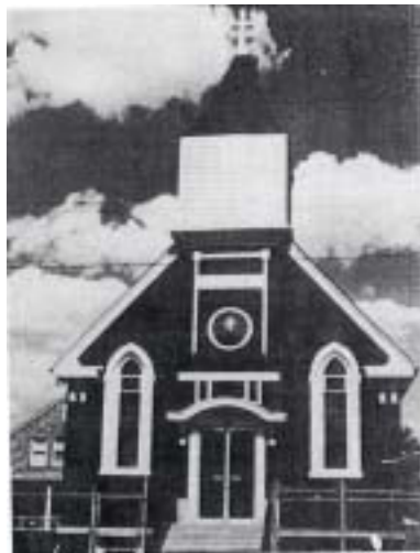
Figure 15 St. John the Baptist Church 9129 Burley Avenue 31
